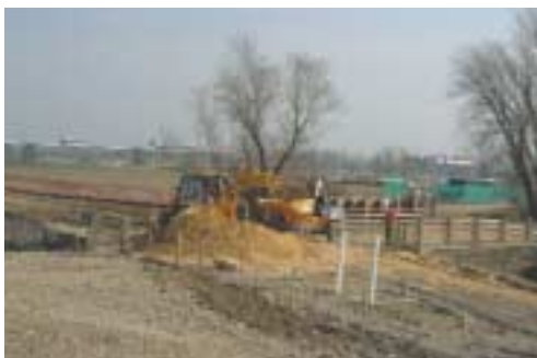
Work beginning on the underground circuits
